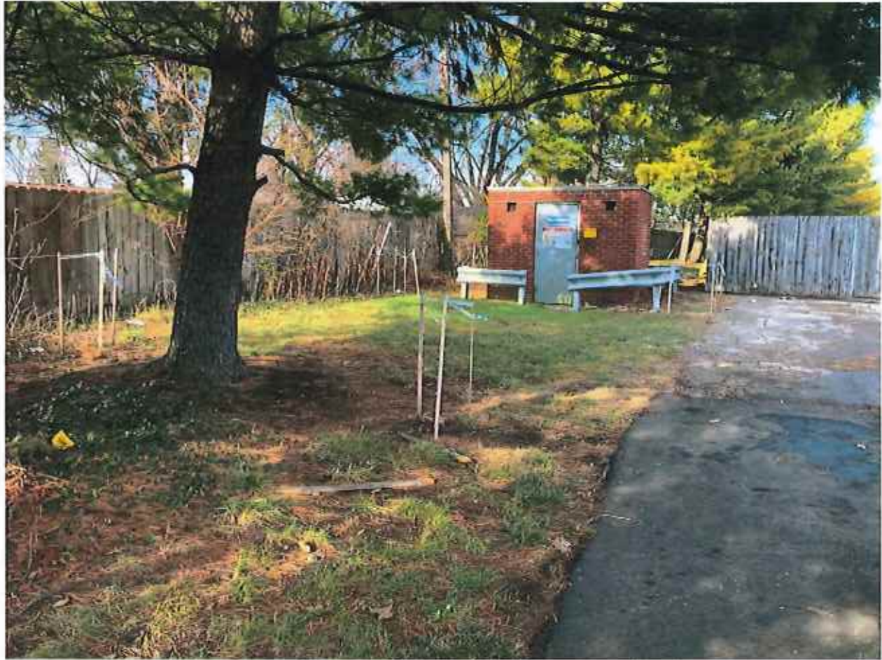
Photo #6: Looking north at typical conditions at Stygler inlet.
